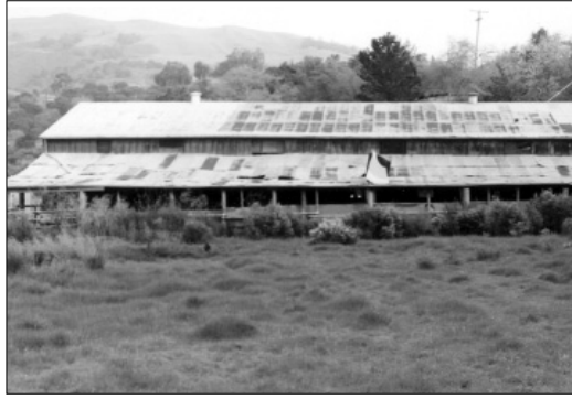
Alum Rock Stables 2003, empty & deteriorating.
